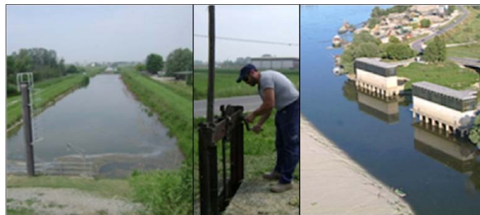
Figure 3 - WATER DISTRIBUTION MANAGEMENT PILOT: OPEN EARTH CANAL (LEFT), MANUAL OPERATION (CENTER) AND WATER INTAKE (RIGHT)
